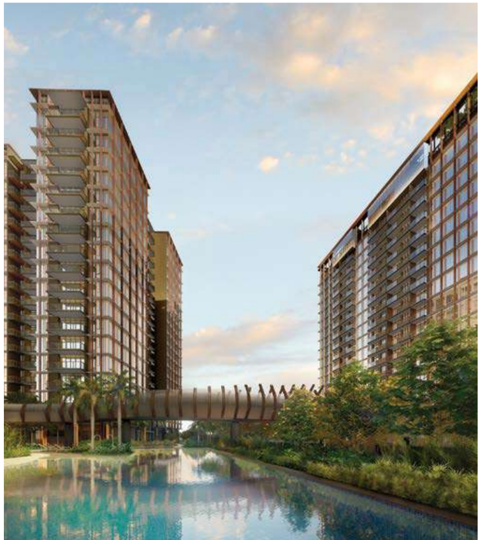
A bridge will link the North and South plots of the development
