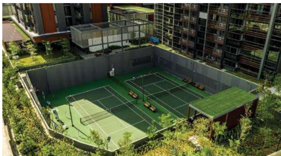
The project has two tennis courts, which are sunken to buffer the noise and so as not to disrupt the view of units on the lower floors
