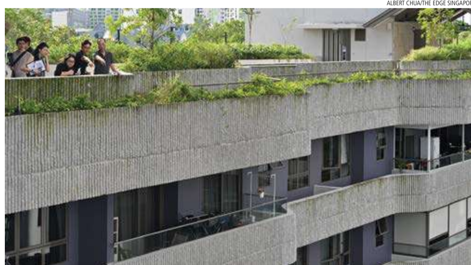
The low-rise residential blocks feature charnfered balconies and articulated brise soleil, creating a unique look
