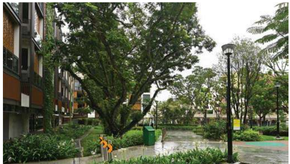
DP Architects designed the project to integrate seamlessly with the public park
