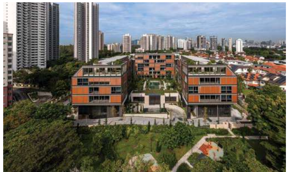
The 56-unit MeyerHouse’s landscaped grounds. They were successfully integrated with the adjacent playground which it had enhanced
