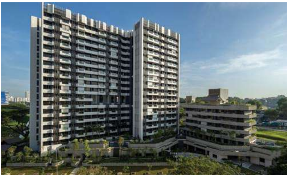
The Tre Ver has multi-tiered landscaped gardens with heritage rain trees and fronts the Kallang River
