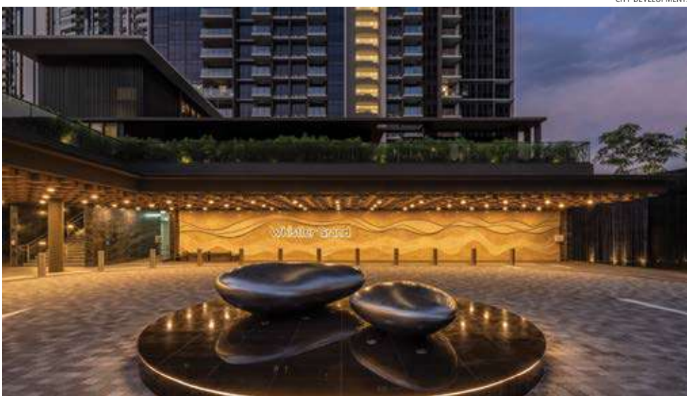
The arrival and drop-off area with its feature wall of black forest stone slabs with matte leather finish
