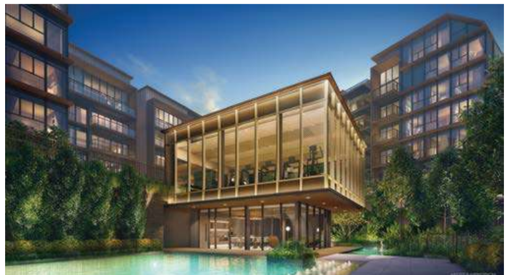
The project was designed by architectural company P&T Consultants with biophilic principles in mind
